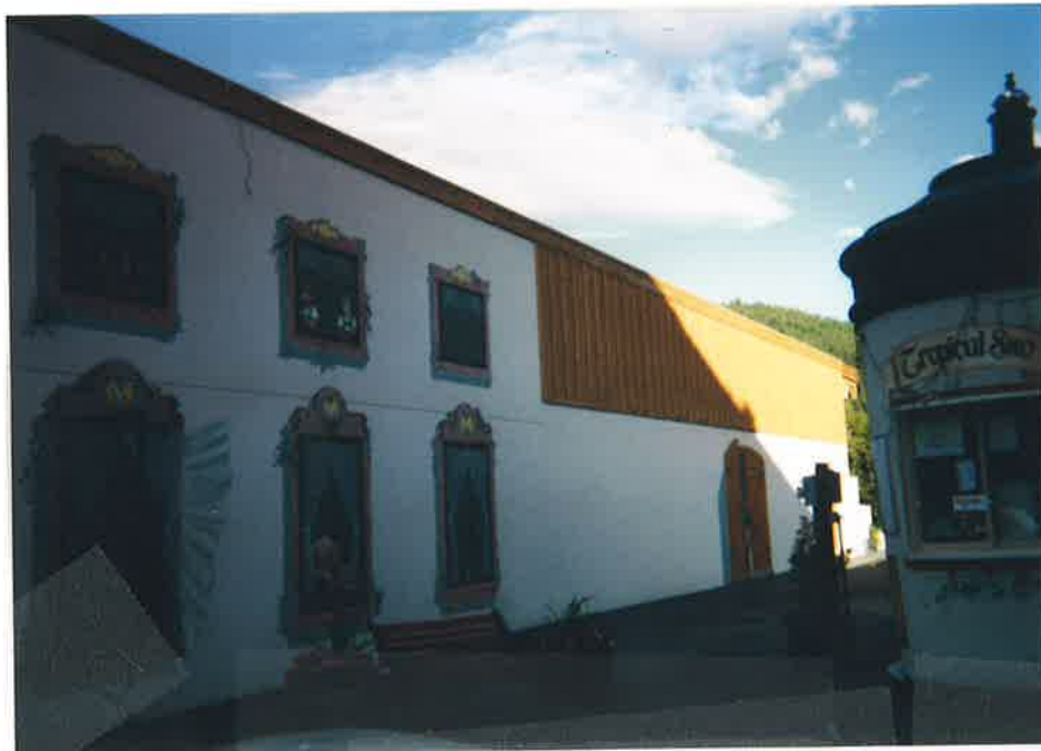
View of alley between two buildings. Because of a narrow alley a roof overhang was not allowed by building code. Notice the paintings of windows on the building on the left breaking up a large area of stucco.
